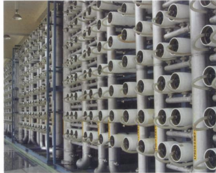
Nanofiltration and low pressure reverse osmosis system at Caotan water treatment, Kaohsiung County, Taiwan. The increasing interest in the effect of micropollutants on the environment and human health will require further treatment processes to be developed. Credit: KINTECH Technology Co. Ltd.
